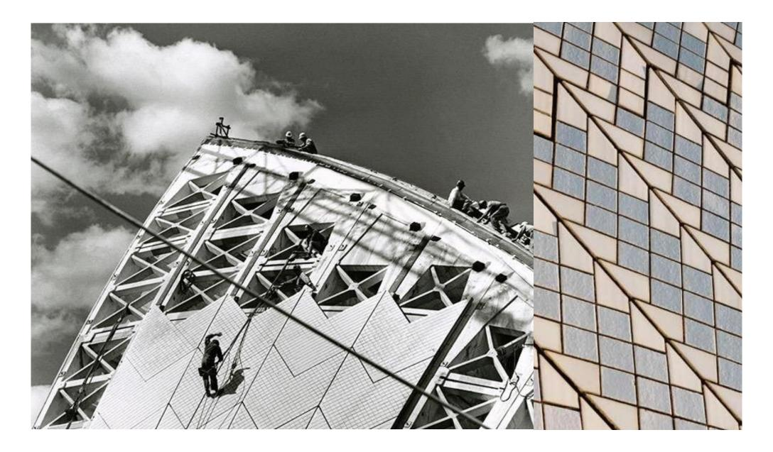
Materials -white and cream mate tiles -precast concrete ribs -steel wire
