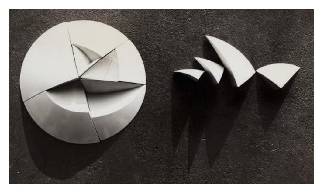
Geometry Spherical solution: Shells as parts of a sphere
